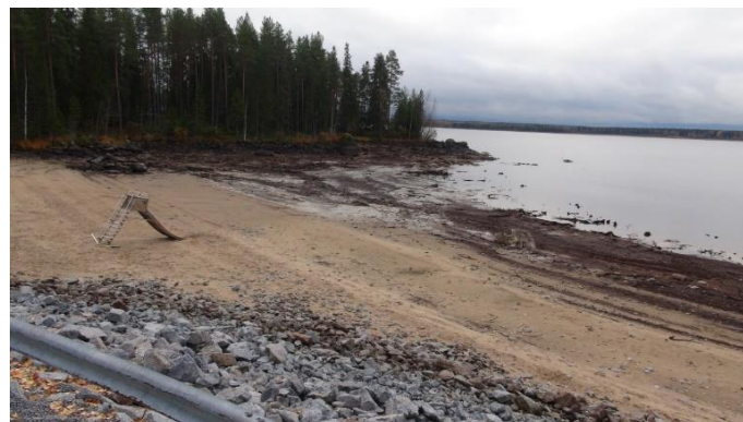
Figure 4.4 - Low water level during 2014 at Hautaperä reservoir.
