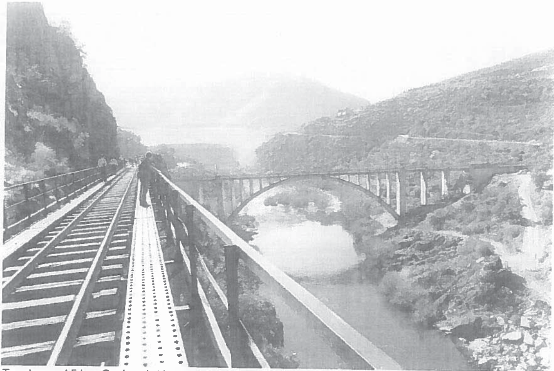
Tua river and Edgar Cardoso bridge, seen from Presas bridge (Construction site for the central plant, on near right, before the bridge)
