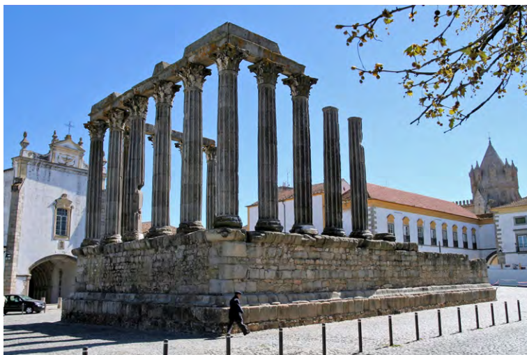
Fig. 11. The Roman Temple of Évora (Portugal) has rich Corinthian capitols of marble topping granite columns, whose bases are also made of white Estremoz marbles (Lopes et al. 2013). On the right can be seen the Cathedral of Évora cupola.
