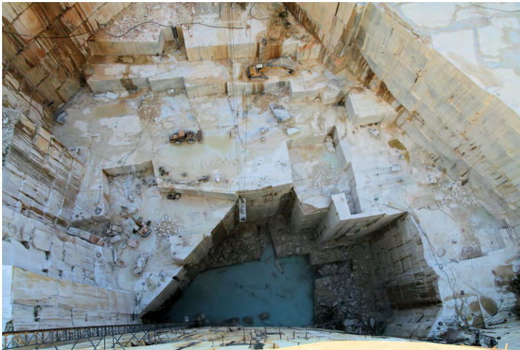
Fig. 7. In the beginning of 2014, the deepest quarry in the Estremoz Anticline was 150 m deep. It is located in the SE periclinal termination of the structure and belongs to F. J. Cochicho Lda. and Cochicho, Lda. companies.
