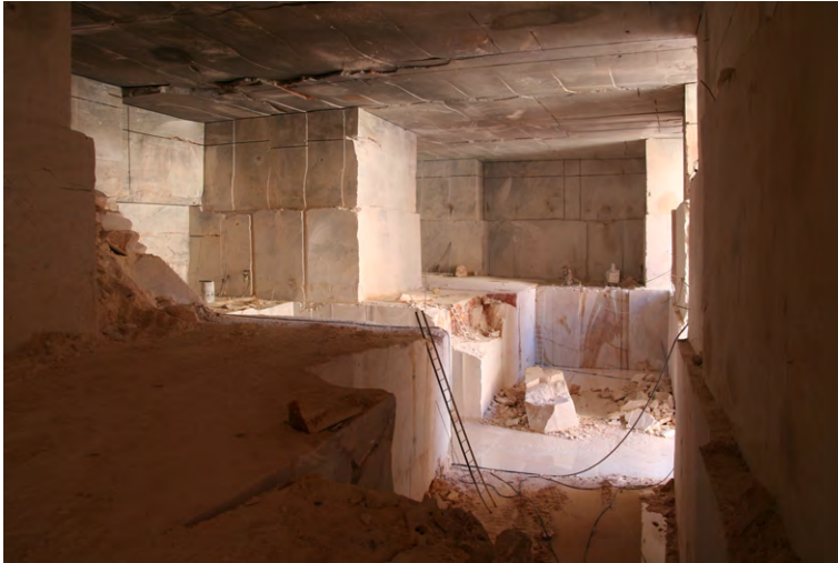
Fig. 8. This image shows the only operating underground marble quarry in the Estremoz Anticline. It is located in the southwest limb of the structure, near Vila Viçosa, and belongs to Lugramar – Sociedade Lusitana de Mármore, Lda company.
