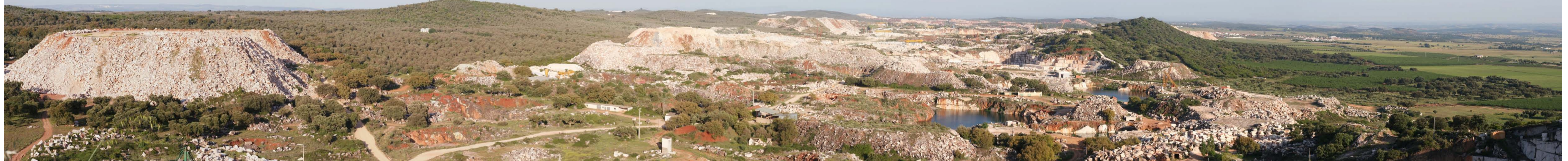
Figure 5. Southwest face of the quarry with the main discontinuities sets: A – open vertical discontinuity associated with karst cavity oriented N-S; B – planar discontinuity with orientation 50/072. The masses highlighted in gray are to be removed. This quarry is located at point 1 in Figure 1.
