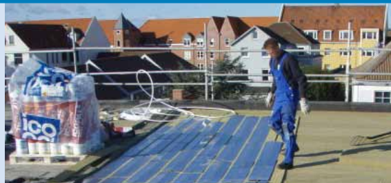
Frederikshavn Police Station has undergone a comprehensive energy retrofit in the insulation of its roof.
