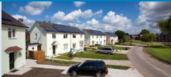
Petersfield – the rehabilitated houses showing solar panels
