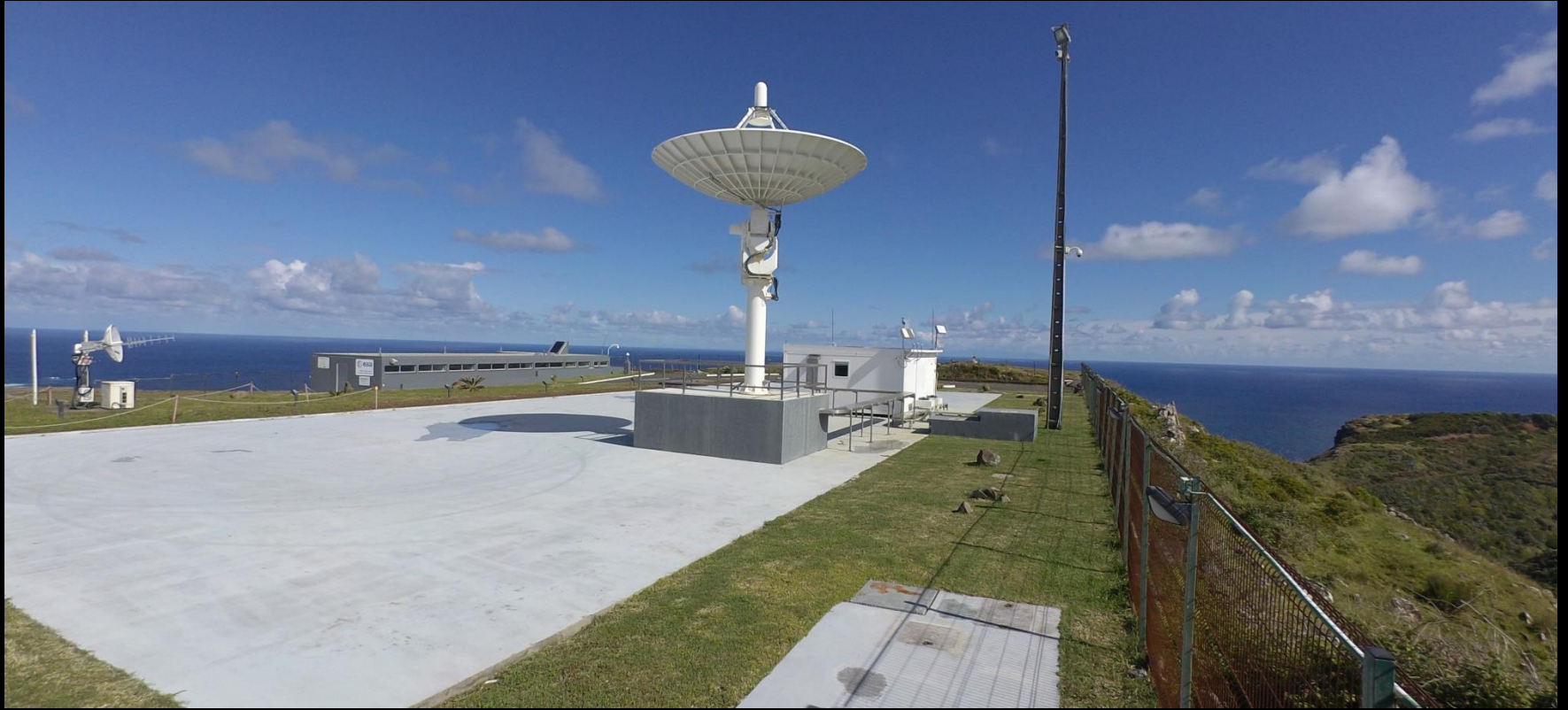
Santa Maria Azores – ESA Tracking Station Operated by EDISOFT since 2007 ESTRACK Stations Network Tracking Station part of Ariane Tracking Stations Network
